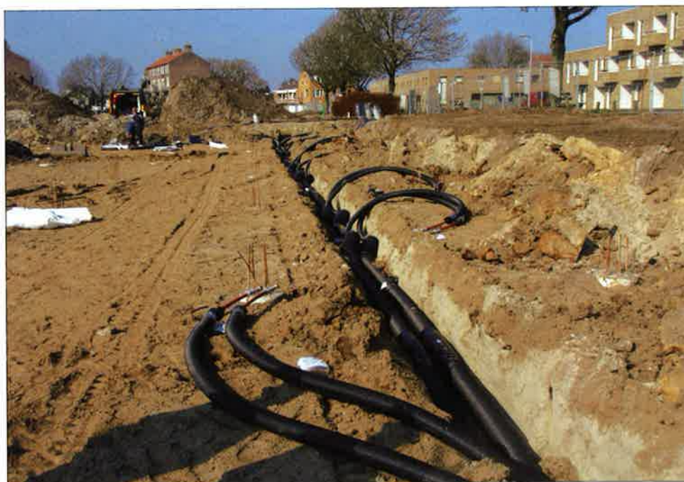
Figure 3. Pre-fabricated systems: laying Flexa Link
