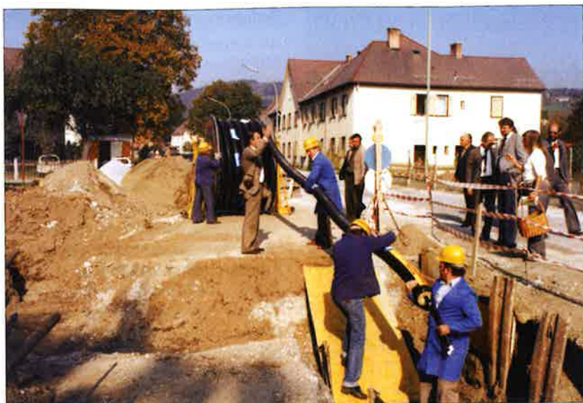
Figure 1. Flexible plastic systems: the first Flexalen installation in 1981
